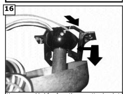
Hang assembled fan from the mounting bracket installed to ceiling in previous step. Make sure the fan is hanging straight. Rotate fan until the tab on the Mounting bracket engages the slot on the Downrod Ball. This must be done to prevent the fan body from rotating when the blades are in motion.
